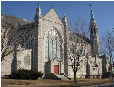
Holy Name Church was built in 1925. It is a National Historic Register building that is significant to the Civil Rights movement in KC. It is currently in disrepair and in danger of demolition by neglect.
