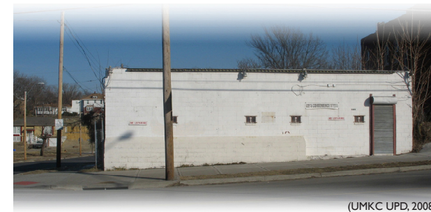
Vacant Commercial Structure at 24th & Prospect
